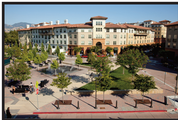
AvalonBay Town Square - 1001 Harvey Drive
